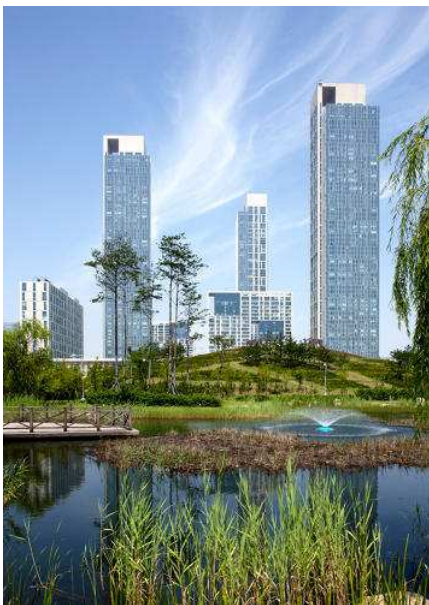
Stormwater is captured on green roofs and also used to irrigate parks.
