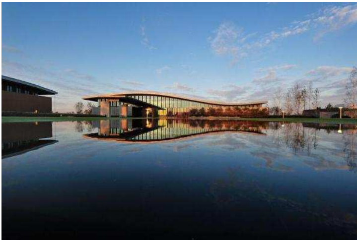
By 2020, the city plans to recycle 40% of the water used;effluent from buildings is used for flushing toilets and street cleaning.
