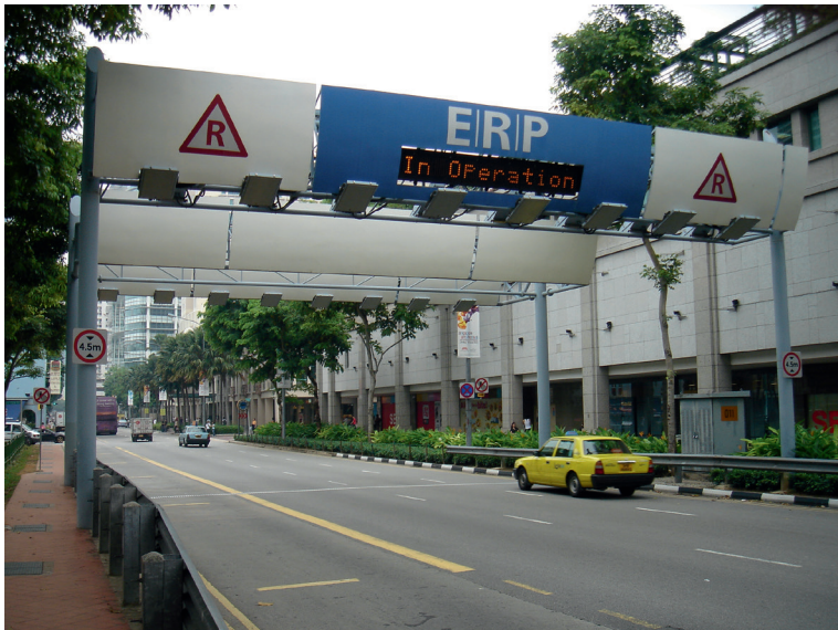
Electronic road pricing gantry in Singapore, 2005 Road pricing to regulate automobile traffic in congested metropolises has become common. In Singapore, vehicles are identified by an electronic device known as an In-vehicle Unit. In Stockholm, where a congestion tax has been implemented permanently since 2007, identification is based on automatic number-plate recognition.
